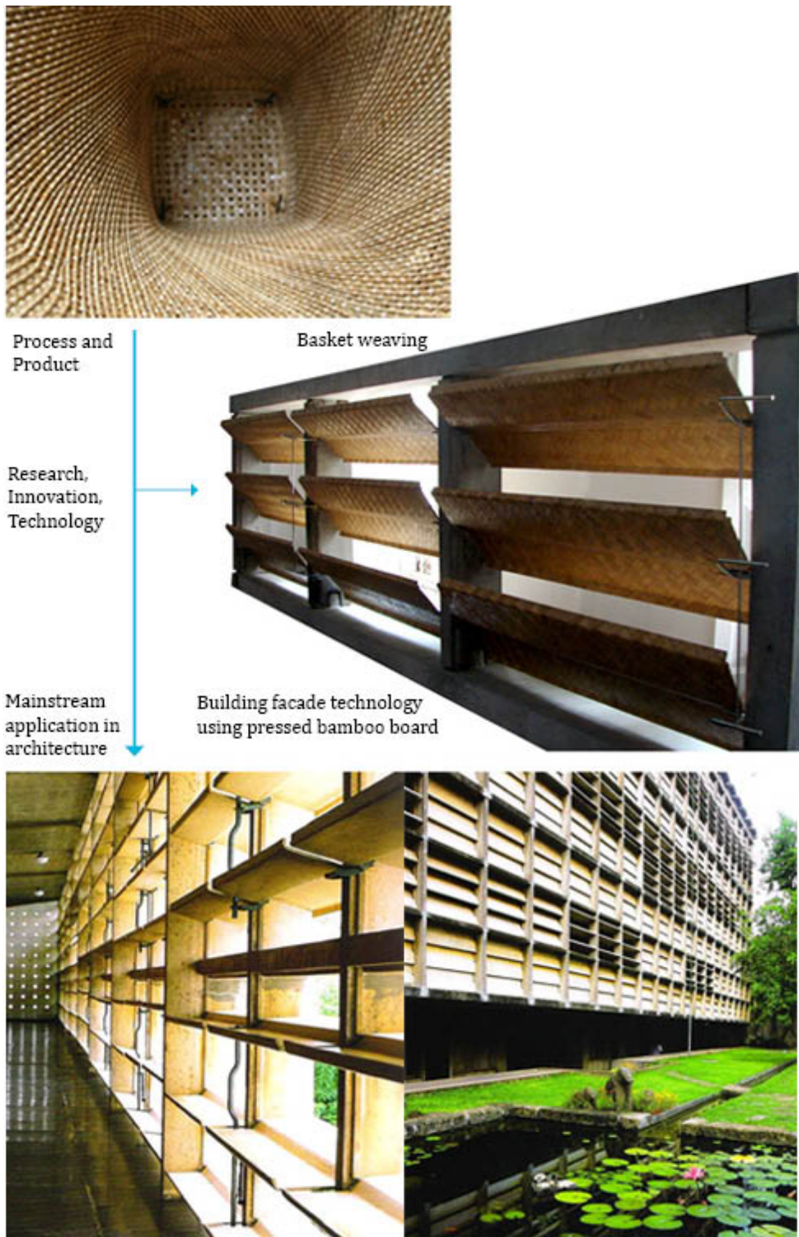
Fig 5: Pressed woven bamboo research for tropical building façade technology, Bangalore This building technology development project leveraged traditional bamboo basket weaving and timber louvers to develop a low-cost building façade technology for mainstream use
